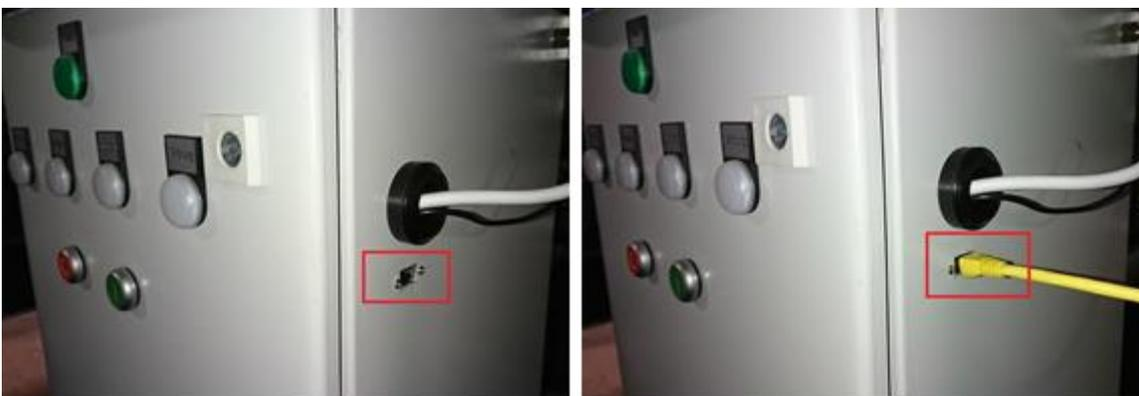
Figure 7: calibration unit Ethernet socket
